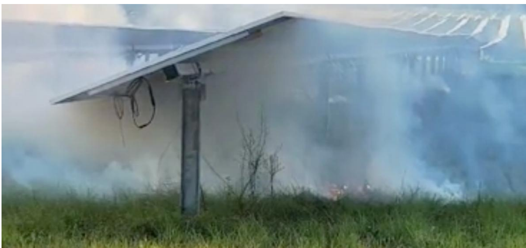
Figure 36: Onsite grass fires, likely triggered by an arc fault, generate dense smoke that can soil and penetrate a PV system, potentially creating long-term reliability risks.
