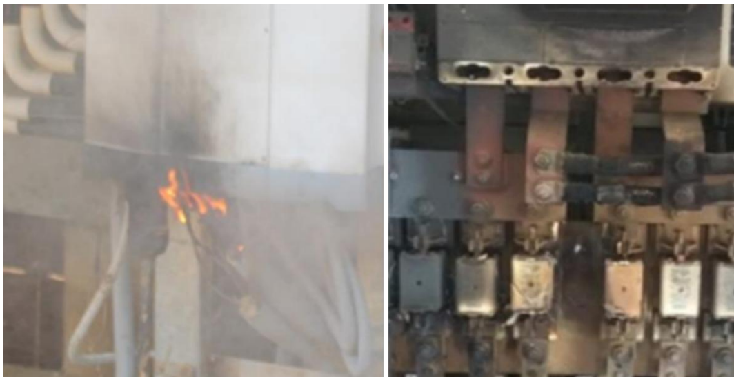
Figure 32: Fire at the inverter and burned SCB at a flood-affected PV plant.
