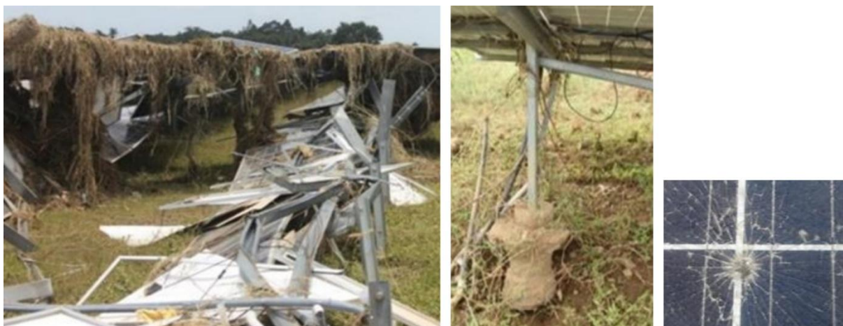
Figure 29: Damage to PV structures due to fast-flowing flood waters in southern India. Examples include destroyed modules and structures; uprooted foundations; and broken glass hit by waterborne debris.
