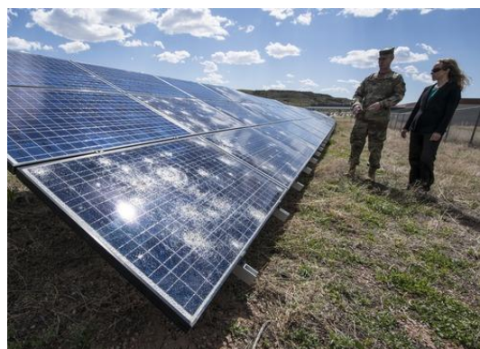
Figure 9: Solar array in Colorado damaged by a record hailstorm that impacted 25–50% of the on-site PV modules. Photo: Dennis Schroeder / NREL.
