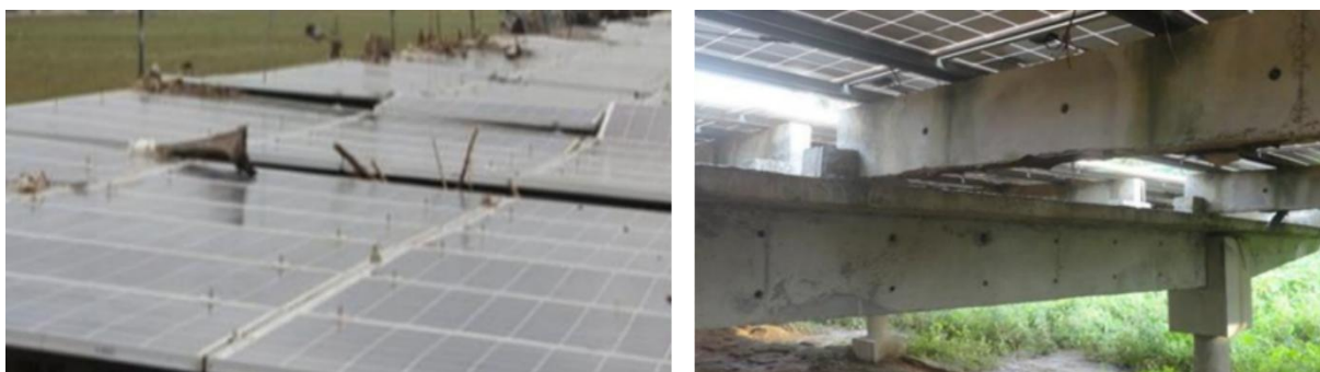
Figure 30: Canal-top PV system with concrete structures proved resilient to flooding because the low-tilt design posed less resistance to the fast-flowing water.
