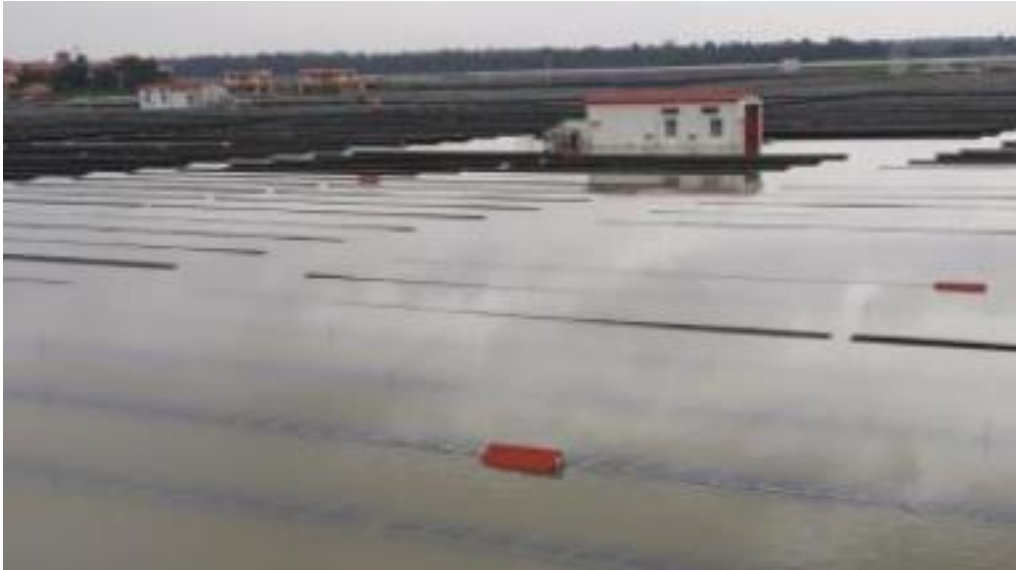
Figure 31: Parts of a PV plant are submerged in 1-3 feet deep water for about two days during a flooding event.
