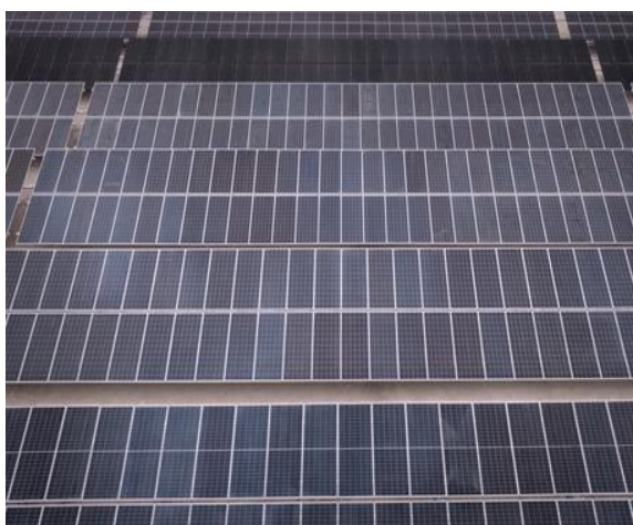
Figure 14: Overview of SOLARCYCLE’s second-life PV installation, made of retired PV modules, after evaluating their residual power output. Bottom-right photo of the PV1 array of the installation, shows example of reused PV module with broken glass, that is still producing energy.
