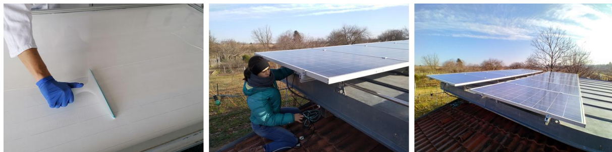
Figure 6: Foto of the coating process of an aged module with cracked backsheet (left), on-site material and adhesion tests (middle) and of the test-site operating successfully with repaired/coated PV modules since 2021 (right). As repair coatings flowable silicone and a two component Polyurethane-coating were used [10,11,33].
