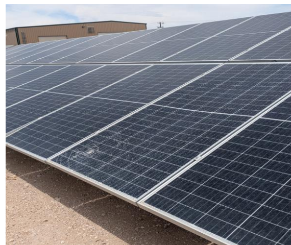
Figure 14: Overview of SOLARCYCLE’s second-life PV installation, made of retired PV modules, after evaluating their residual power output. Bottom-right photo of the PV1 array of the installation, shows example of reused PV module with broken glass, that is still producing energy.
